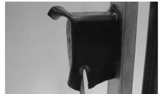
Step 4: Adhere remaining pad to box and cut to provide a snug fit around conduits or cables.
