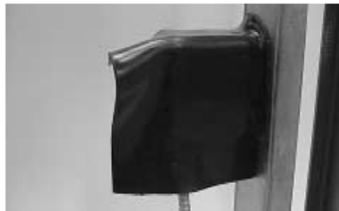
Step 3: Starting at top, align to front edge of box and overlap onto the stud 1/2 inch (13 mm).
