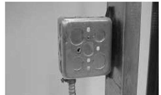
Step 2: UL Listed metallic or nonmetallic outlet boxes (refer to above listing)
